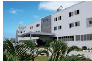
Rudrapur Plant (Green Building)
